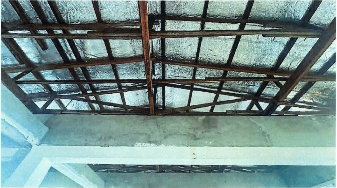
Figure 18 No major defects seen in roof structure
