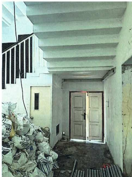
Figure 19 No defects seen in stair structures.
