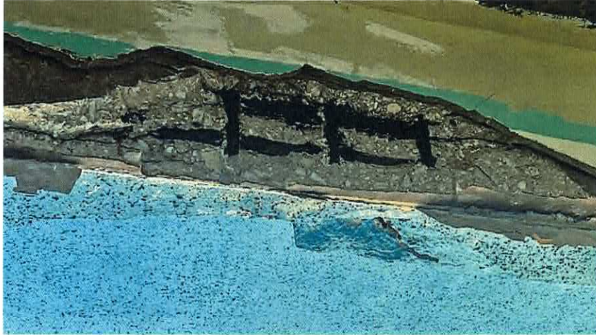
Figure 7 RC Beam spalling damage, 1st floor
